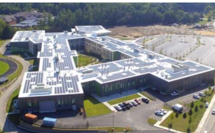
City of Dover Dover High School, Indoor Pool, CMNH 1 MW (2018-9)
